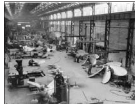
Manufacture of propellers at the Nantaise de Fonderies in 1950-1960.
